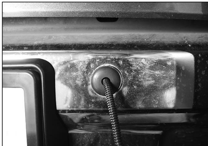
(Fig 16) Models with sensors, slide Grommet over small end of Harness Extension. Push Grommet into hole in bumper and attach to wiring harness
