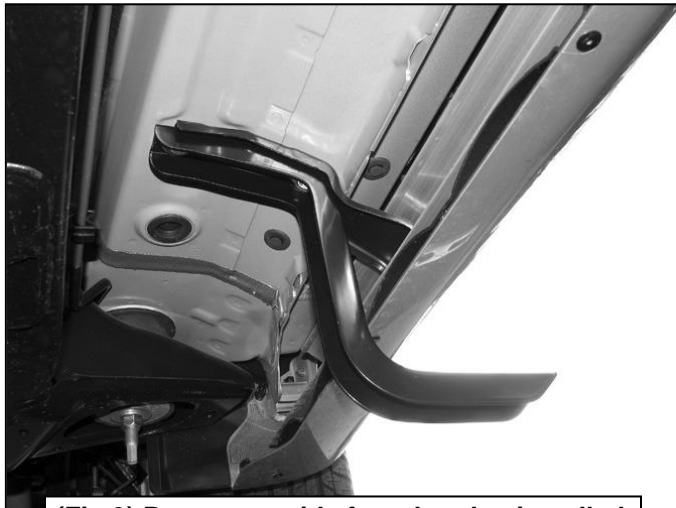
(Fig 3) Passenger side front bracket installed
