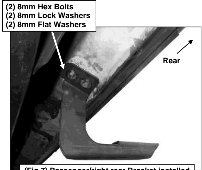
(Fig 7) Passenger/right rear Bracket installed
