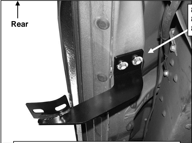
(Fig 5) Driver/Left Rear Bracket installed
