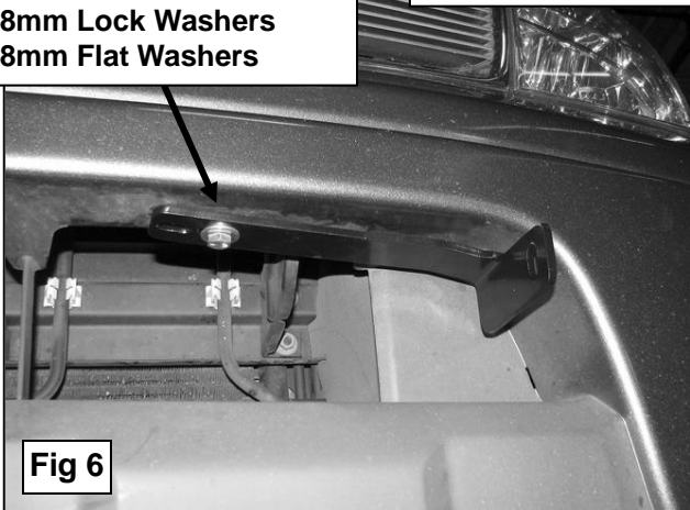
05-08 driver side Top Bracket installation pictured
